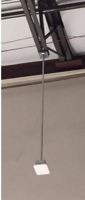
Installed Drop Pole Assembly
